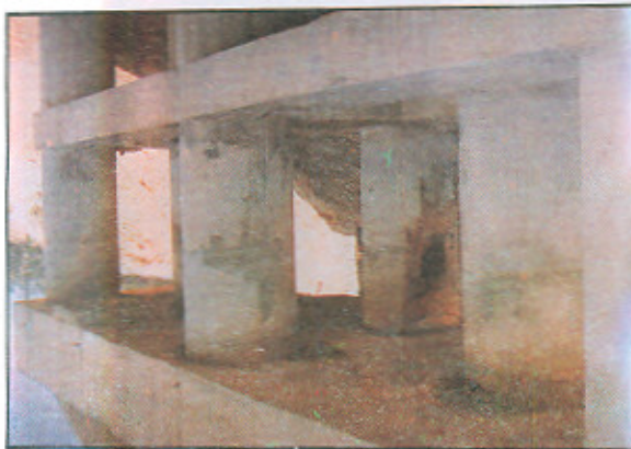
Fig.3 Hi-Bond has been effectively used as an admixture to RCC for cladding and pile strengthening of cracked piles in earthquake damaged Bridge at Lora Nallah, Brewery Road, Quetta. (a) Mixing of Hi-Bond with the mix, (b) Pile strengthening with additional re-bars, (c) Appearance of piles after cladding. (Courtesy: M/s Loya Associates, Karachi)
