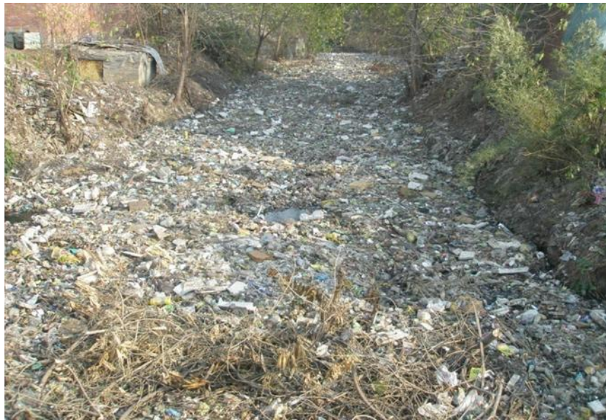
Fig. 4: Shadman drain carrying sewage and solid waste in to the Ravi
