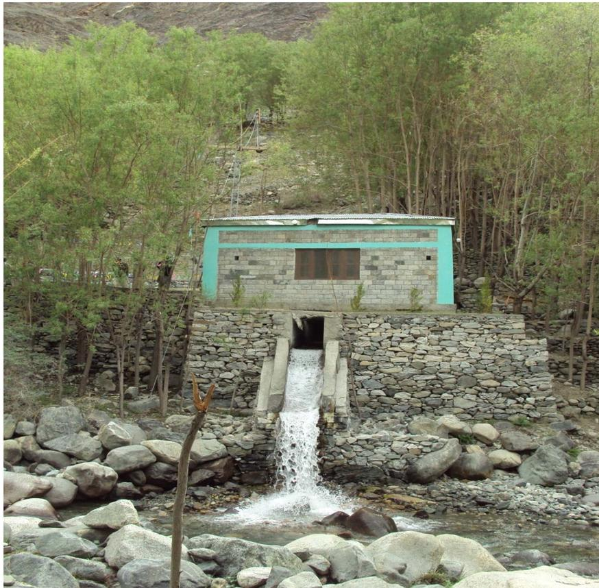
Fig. 2 View of Power House water back into nullah after generation of Electricity.
