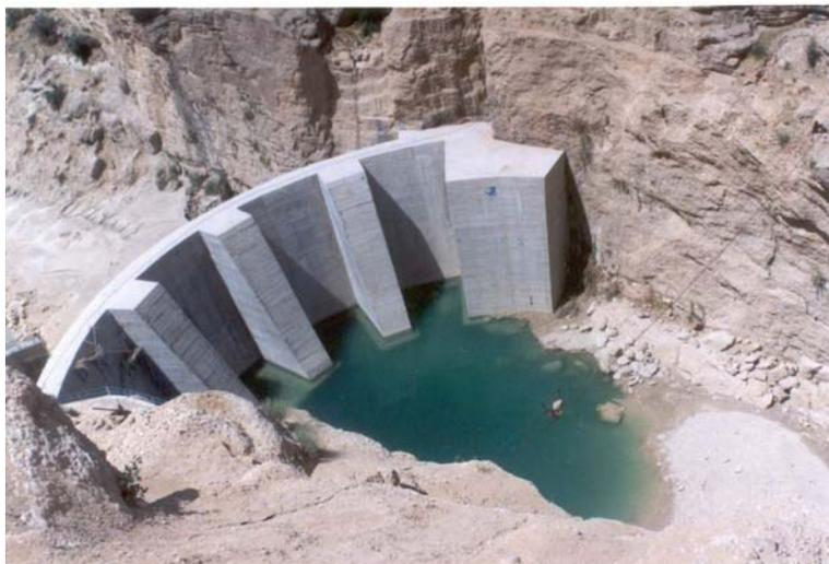
**Figure 5:** Delvari Cofferdam after the second overtopping (April 2002)
