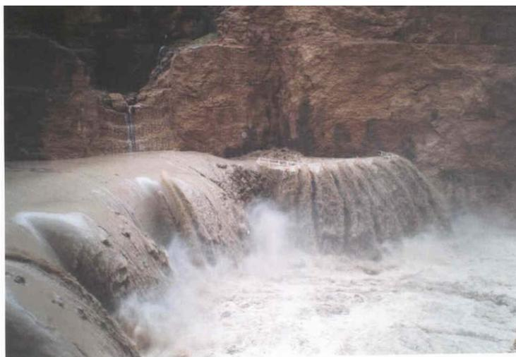
**Figure 4:** Overtopping of Delvari Cofferdam to maximum height of 4.7 m (Jan. 2002)
