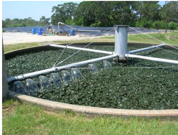
Fig: 4 Waste water Treatment by Tricking Filter.
