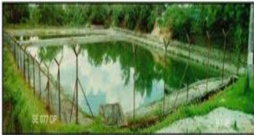
Fig: 7 Algae-based Waste water Treatment
