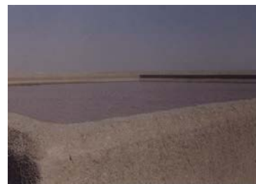
Reservoir with Filtration Plant
