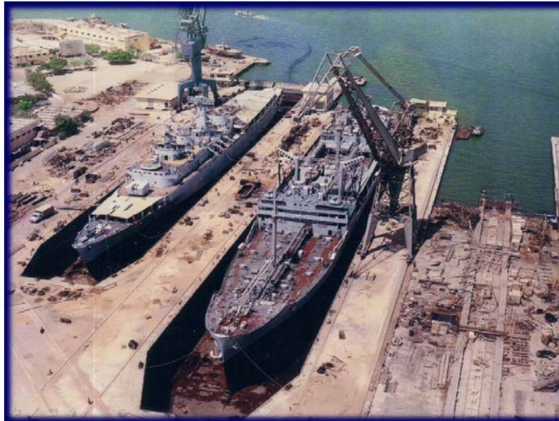
Ships under repair at Dry Docks
