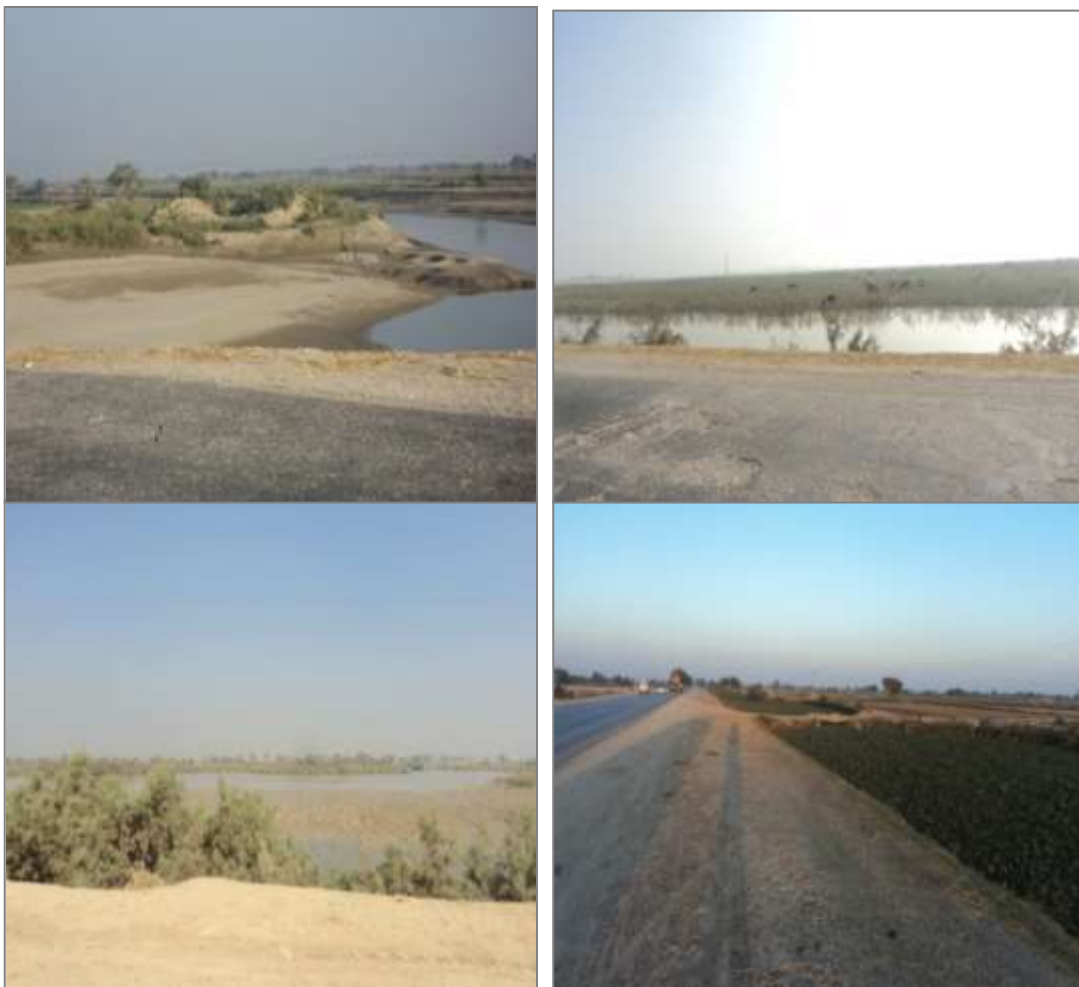
Figure 5: Upper left-Sindh Feeder crossing Shikarpur-Kandhkot road, oblique crossing is de-routing the channel; others showing standing water - Shikarpur-Kandhkot road.
