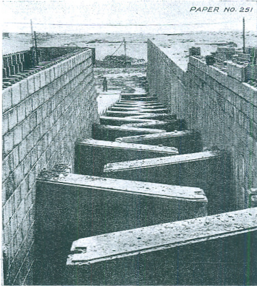
FISH LADDER ALONG THE LEFT DIVIDE WALL UNDER CONSTRUCTION (June 1941)
