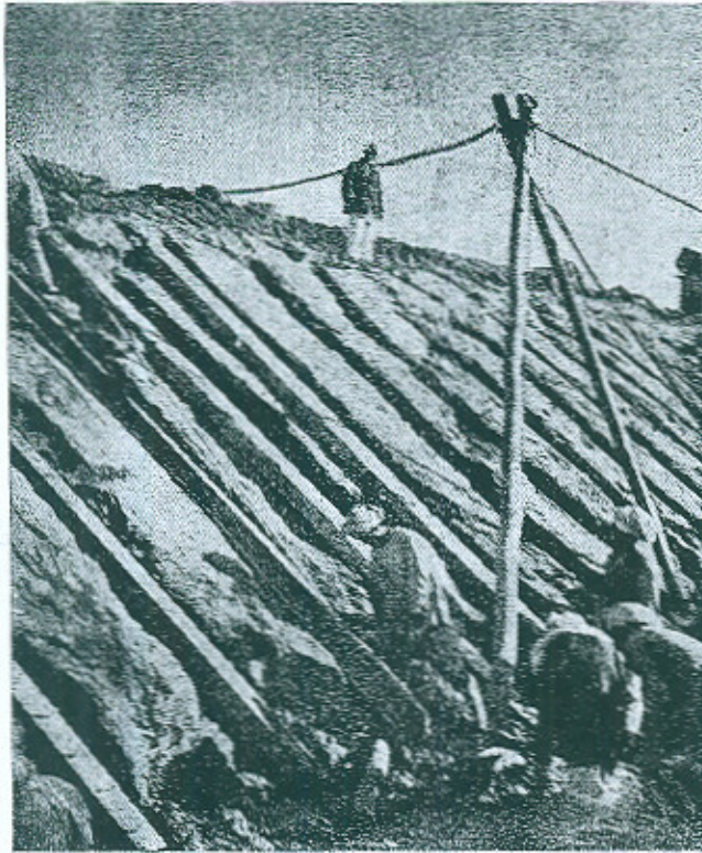
Laying, spacing and aligning beam.
