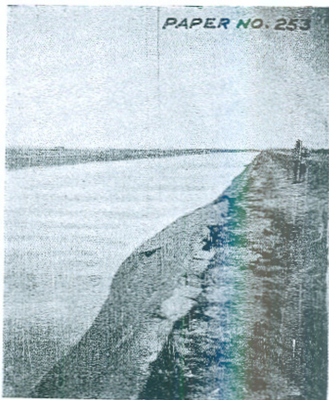
Note the drain cut behind the lining and marks of wave action.
