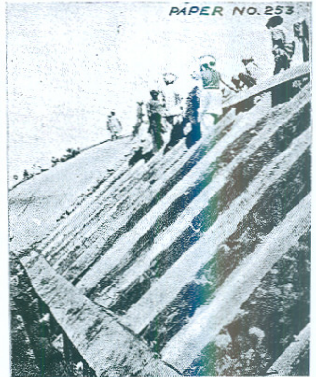
Laying, spacing and aligning beam.
