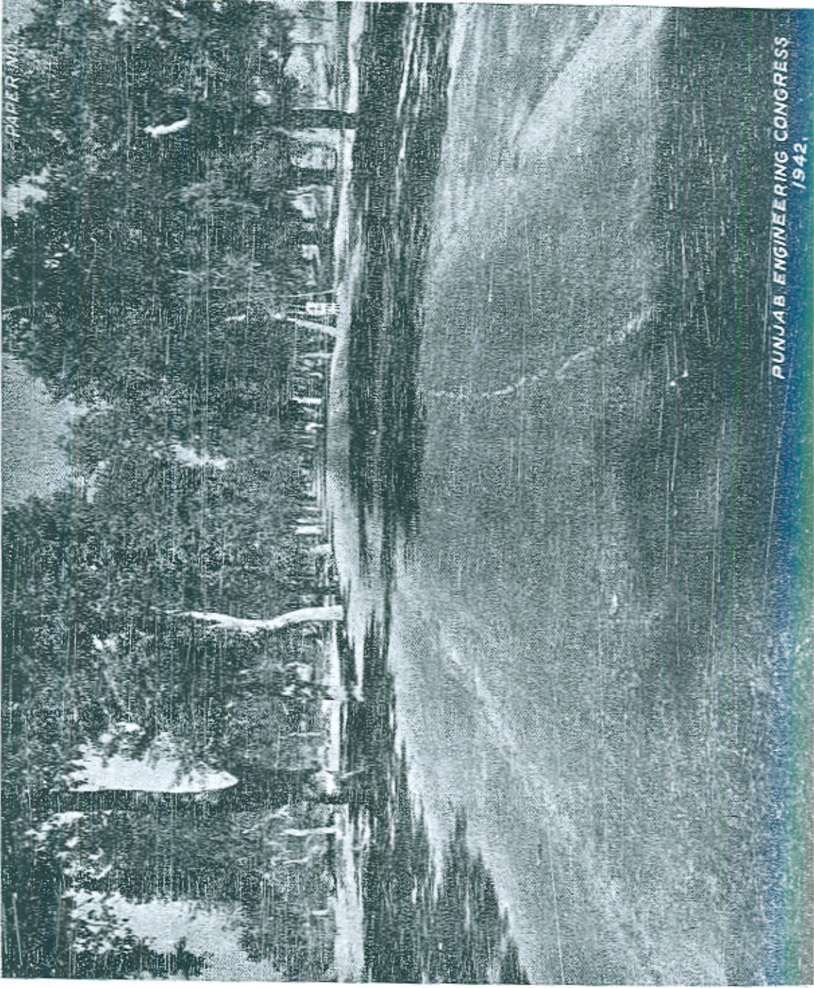
FIG. 10 EXPERIMENT IV—BERM STABILIZATION ON LAHORE-FEROZEPUR ROAD. STATE OF THE BERMS SIX MONTHS AFTER COMPLETION. THE UNSTABILIZED PORTION OF THE BERM IS ALSO IN GOOD CONDITION.
