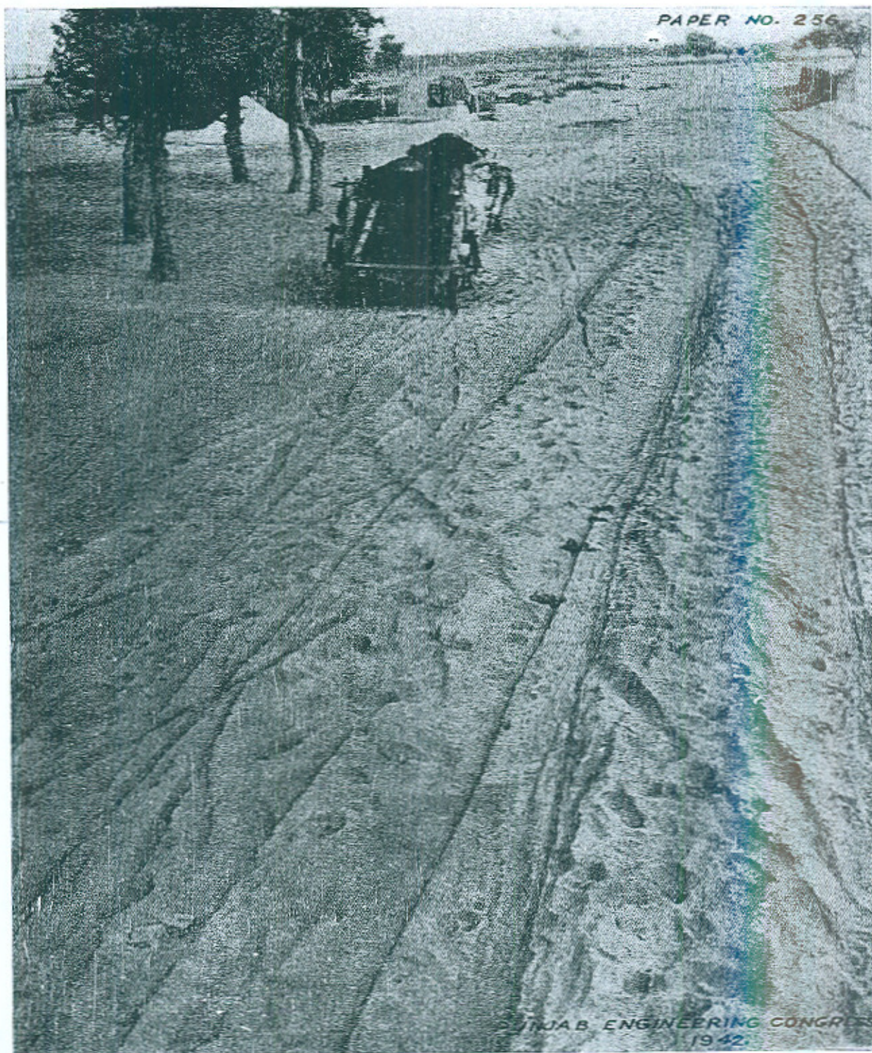
FIG. 1 EXPERIMENT I—KOT LAKHPAT LINK ROAD. SHOWING THE STATE OF THE STABILIZED AND UNSTABILIZED PORTIONS IN THE DRY WEATHER. STABILIZED PORTION IS IN THE BACKGROUND.
