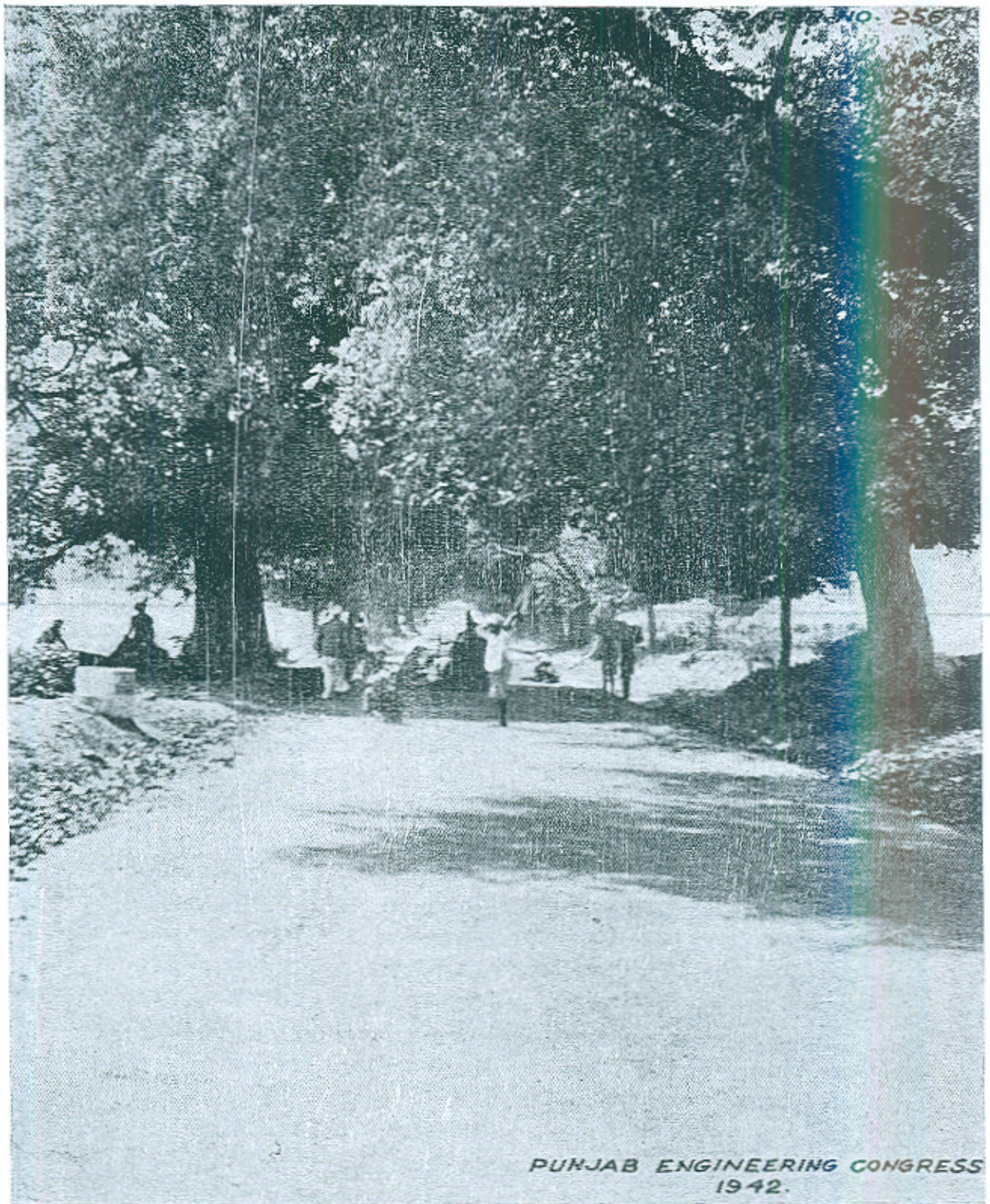
FIG. 6 EXPERIMENT II—HOSHIARPUR-BHARWAIN ROAD, SHOWING THE STATE OF THE STABILIZED ROAD, IMMEDIATELY BEFORE THE COMMENCEMENT OF SURFACING, A YEAR AFTERWARDS.
