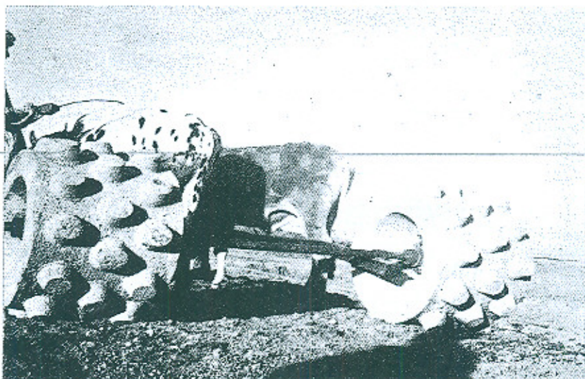
TOOTHED ROLLER IN TWO PARTS WITH A CONNECTING SHAFT
