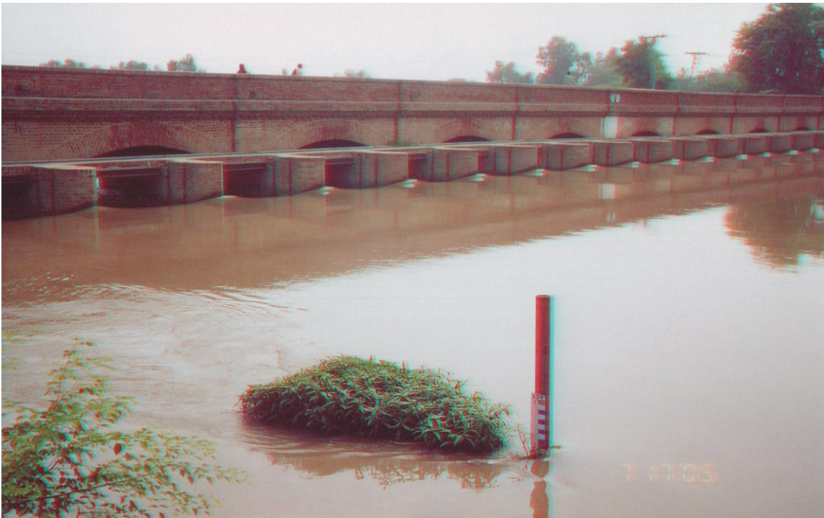
Photo # 4: View of Upstream of Fall RD 59.815 km Main Canal (LBDC)
