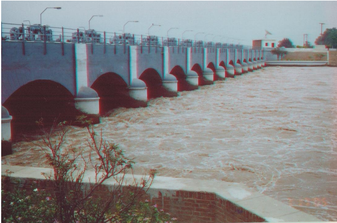
Photo # 1: View of Head Regulator of Main Canal RD 0 (LBDC)
