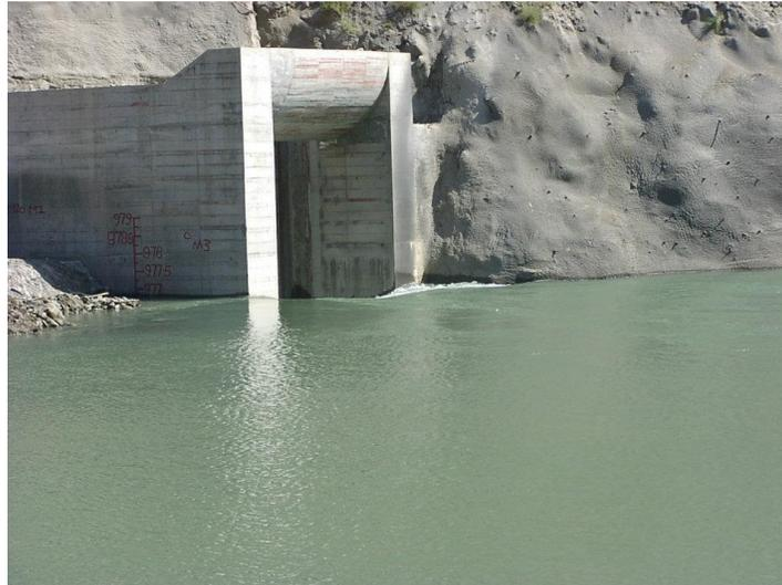
**Figure 5: River Diverted Through Diversion Tunnel On 15 October 2011**
