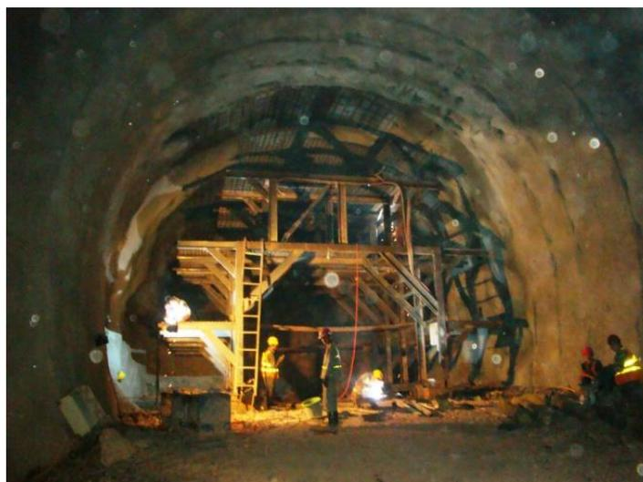
**Figure 4: Excavation of Headrace tunnel**
