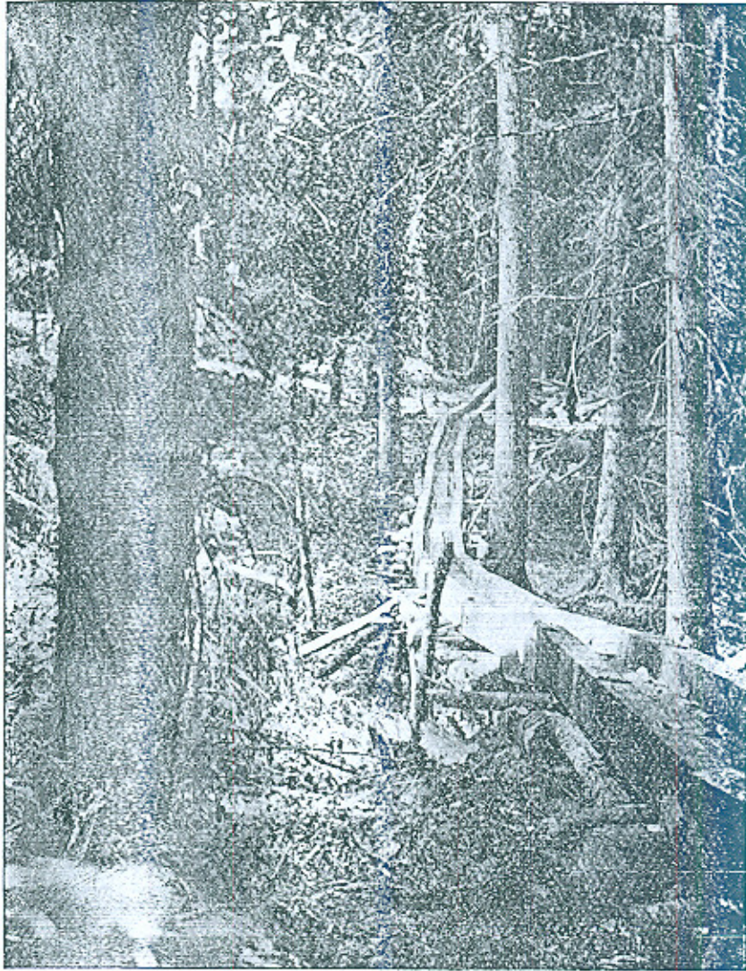
A dry slide for beams 16'×12"×6", the Gaura Forest, Bashahr.
