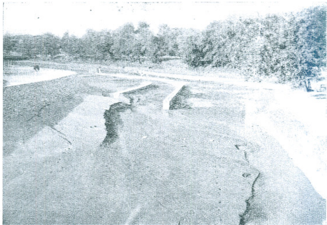
Photograph showing a view of the vanes and the channel upstream of the Salampur Head Regulator. It will be seen from this photograph that a large quantity of silt and shingle is ejected by the vanes.
