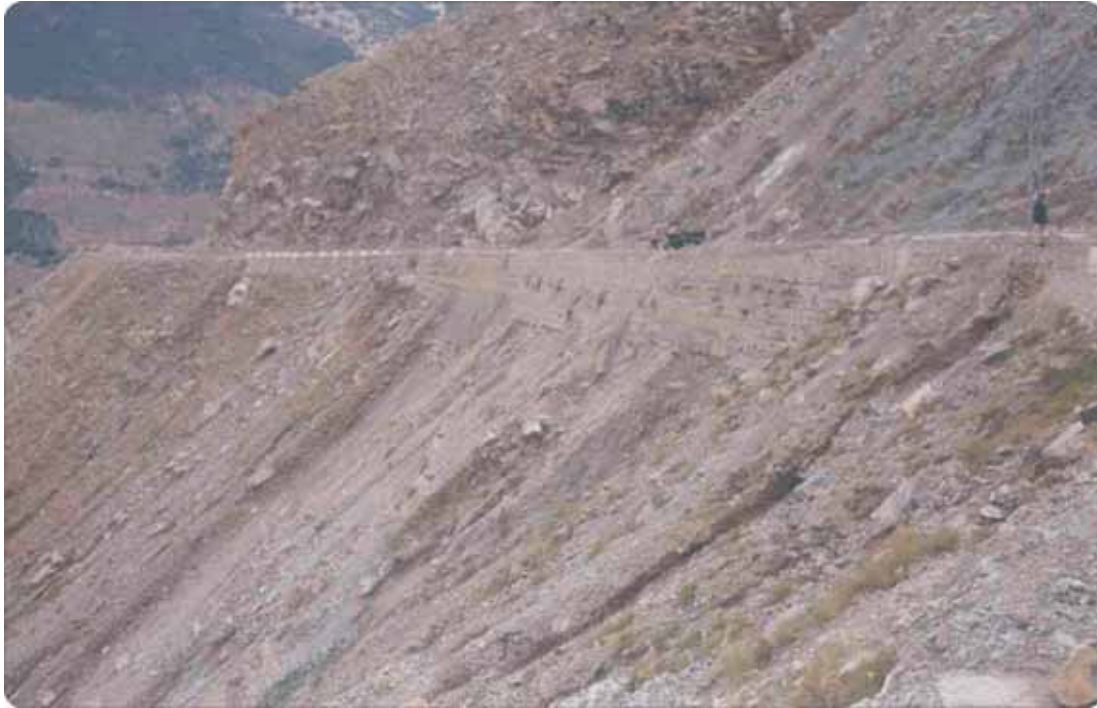
Figure- 6: Another example of scree and debris material subject to sliding on both upslope and downslope portions of Jijal landslide site.
