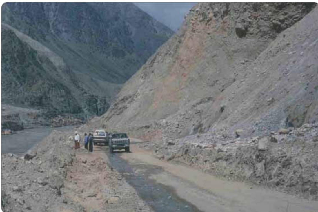
Figure 7: Another view of steep slopes at the Tatta Pani landslide site covered with loose and unconsolidated materials.
