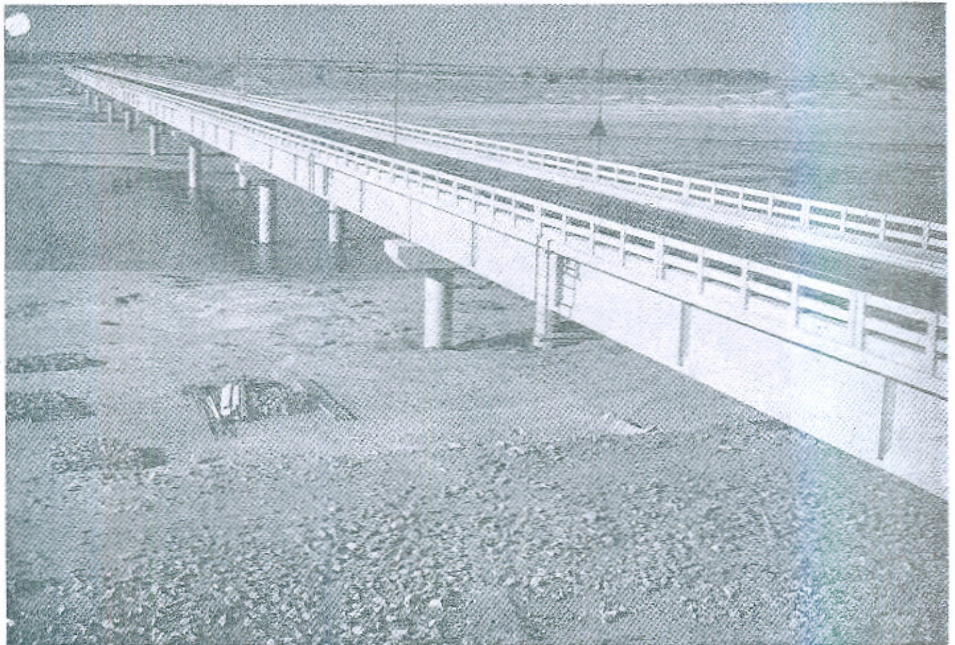
New Bridge over River Sutlej near Bahawalpur
