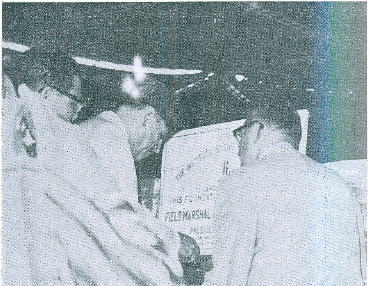
The President laid the foundation-stone of the Lahore Centre of the Institute of Engineers, Pakistan
