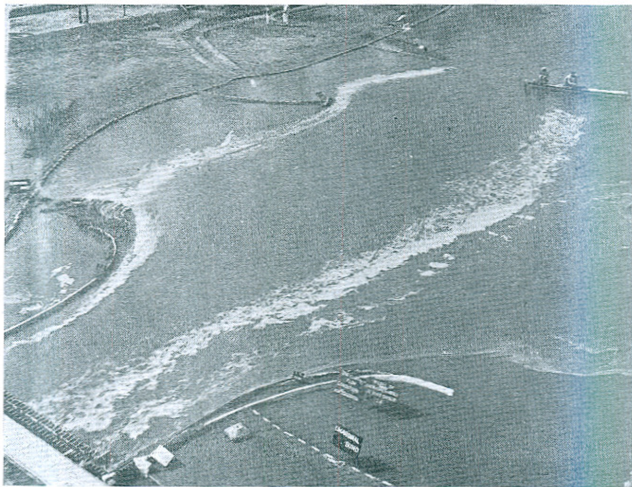
Model of Qadirabad Barrage of River Chenab, Upstream River Training Works
