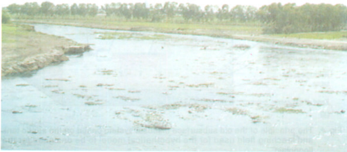
Fig. 2. The high risk piece of land between the sewage channel (outfall) and the active channel of river Ravi proposed for the treatment plant. This photograph was taken in June 2004.
