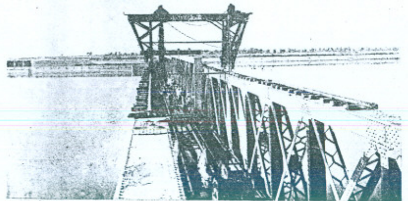
4. CUTTING UP MAIN GIRDERS. SHOWING GANTRY FOR LOADING
