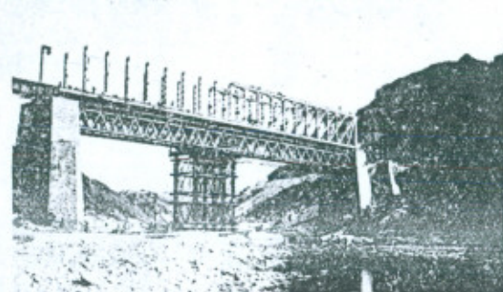
6. ERECTING MAIN MEMBERS OF 250 FT SPAN
