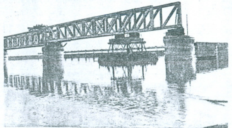
2. SUPPORTING GIRDERS OF DISMANTLED SPAN ON PONTOONS FOR FLOATING BACK
