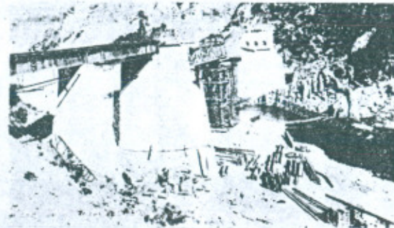
3. ERECTING SERVICE GIRDERS
