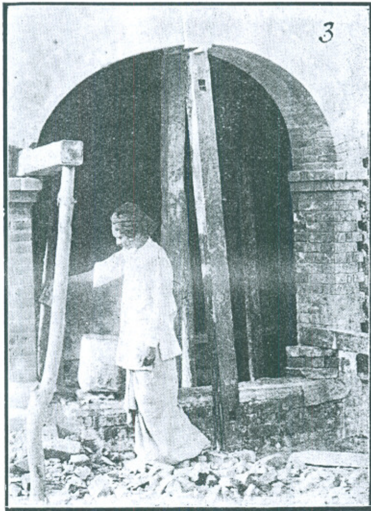
Underpinning of Verandah Pillars.
