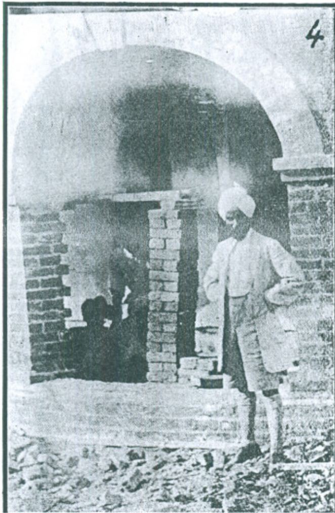
Underpinning of the cross in the front Verandah.
