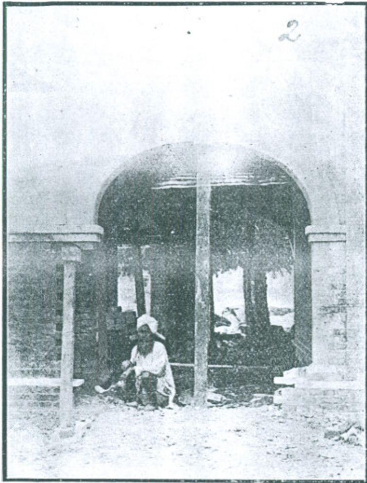
Underpinning of Verandah Pillars.
