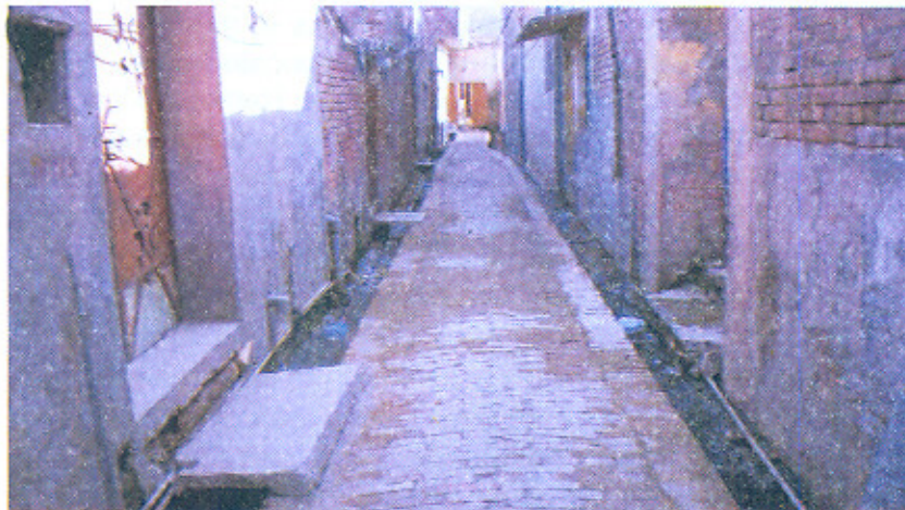
Figure 2 : Open drains in Kotla Arab Ali Khan, Gujrat District
