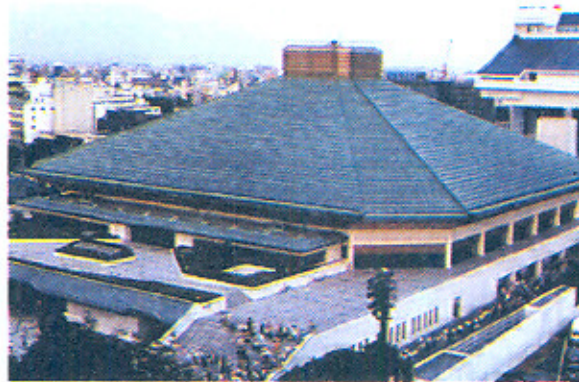
Figure 5: At Kokugikan sumo wrestling arena in Tokyo, Japan, rainwater collected from the arena's 8,400 square meter rooftop is used for non-potable purpose.
